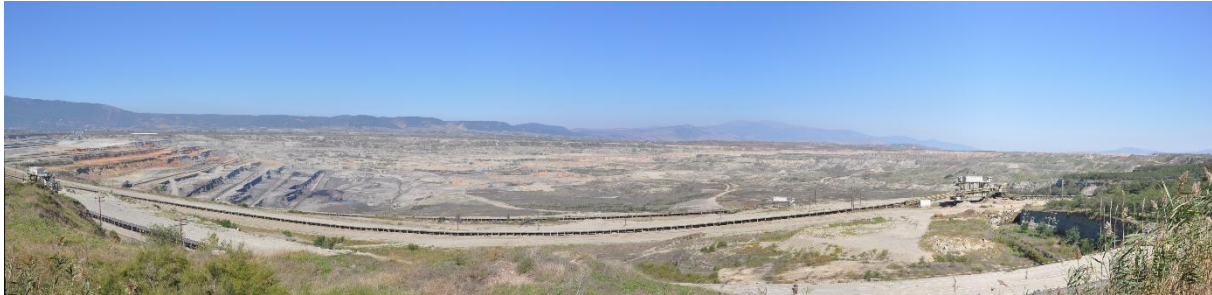
Figure 1 – Overview of the Amynteon strip mine. The largest continuous conveyor is distinguishable in the middle having a length of over 2km.
